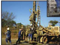
Jobsite photos courtesy of www.wfto.cc
