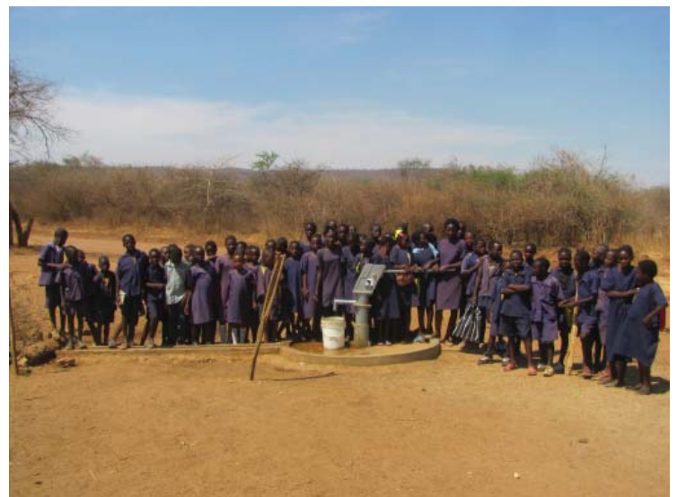
Completed hand pump repair at Kachembele Community School
