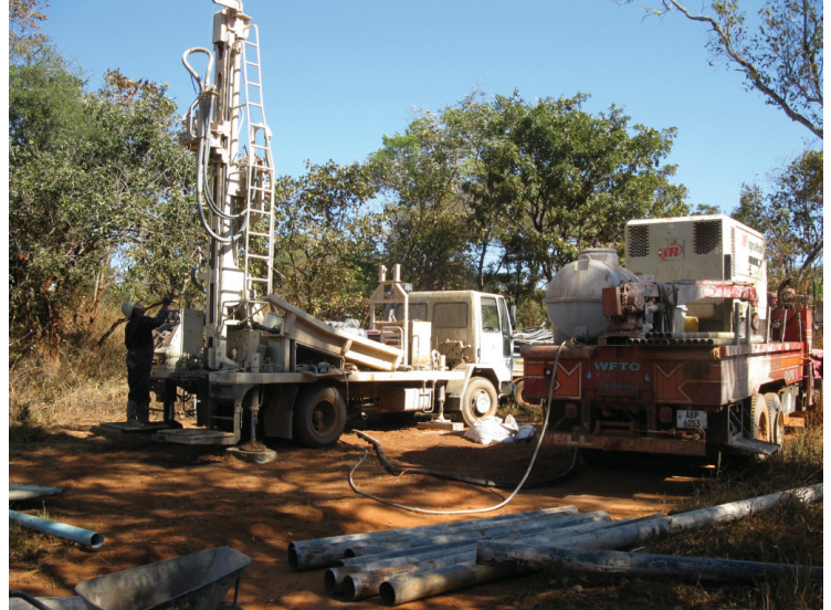
Drilling at Kamfumfula Village
