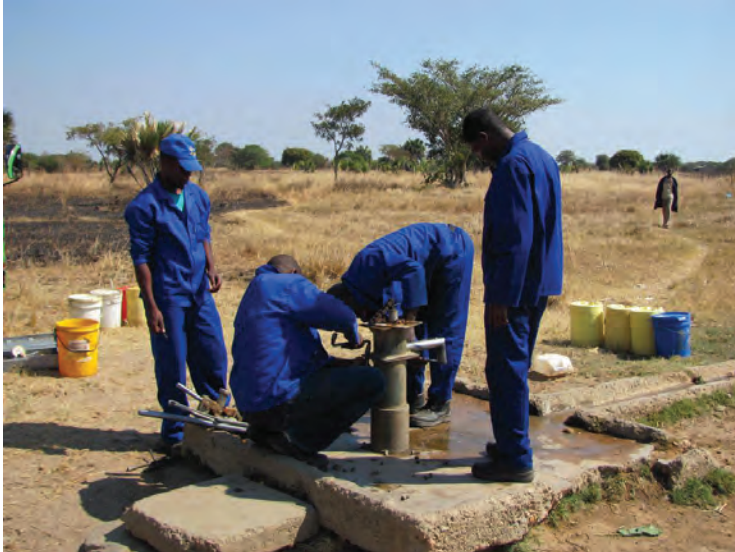
Katenga Village: The hand pump repair is just beginning but the Jerry Cans begin to accumulate as people are searching for water.
