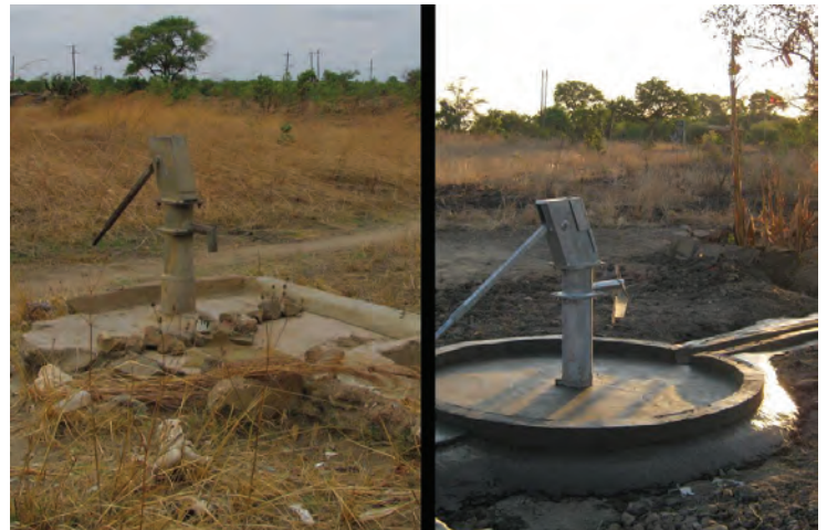
Before and After Hand Pump repair, Mulala Village
